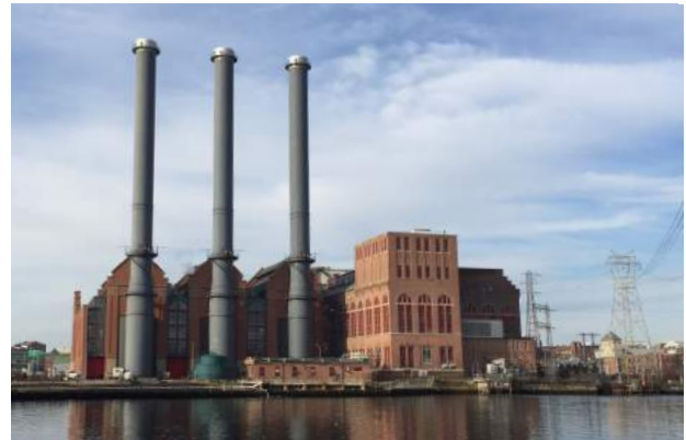
Manchester Street Power Station. Photo Credit: City of Providence.
